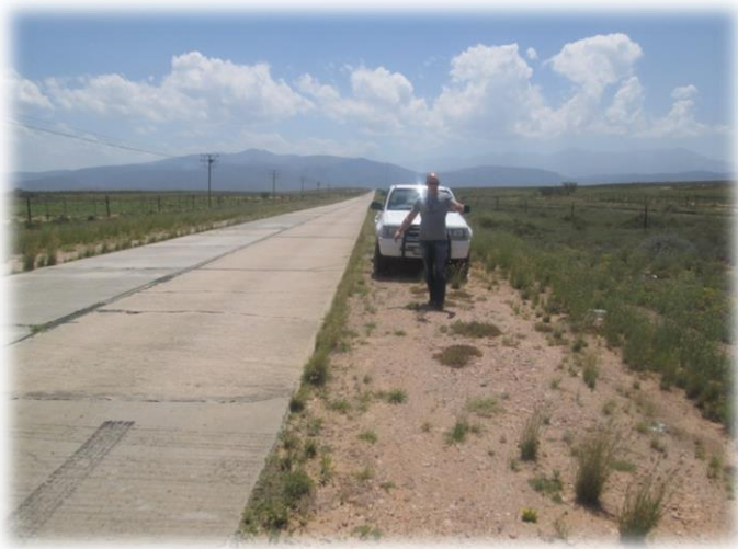
Figure 1: View taken of the compacted road verge/shoulder. This picture indicates more than 2m wide compacted gravel shoulder. The road upgrade activities will remain within the compacted degraded road verge/shoulder. The adjacent plant species towards the fence
