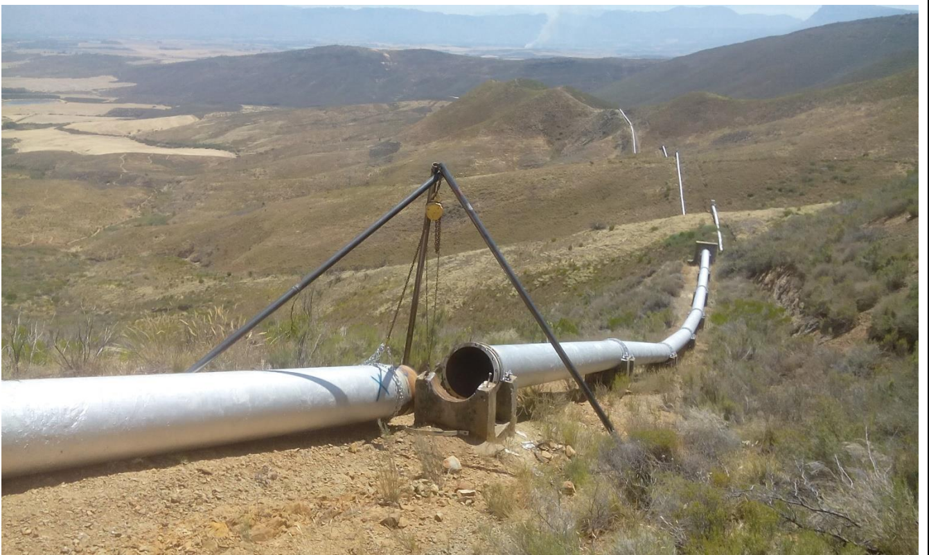
Photograph 4: General view of the pipeline looking north, including removal of a pipeline section for inspection.
