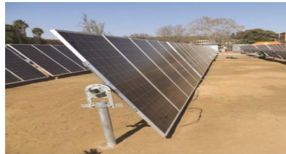
Figure 1: Single axis solar PV module tables raised 500mm above ground level (to a maximum tilt height of 3m).
