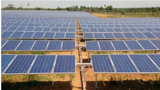
Figure 1: Single axis solar PV module tables raised 500mm above ground level (to a maximum tilt height of 3m).
