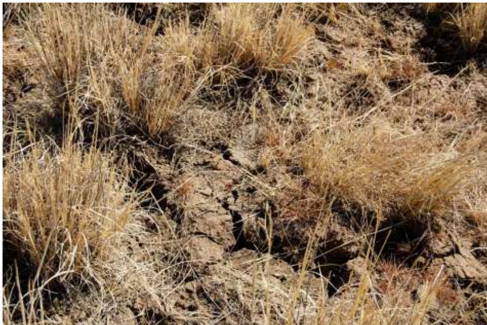
Figure 7 Dry clayey soil with cracks
