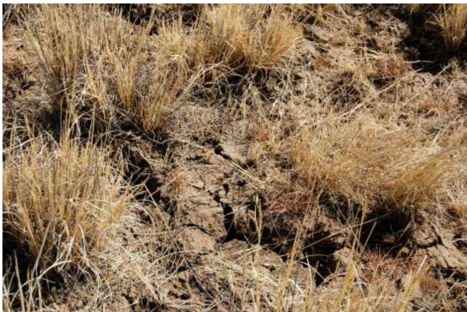
Figure 7 Dry clayey soil with cracks
