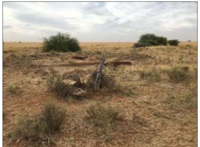
Figure 30. Demolished laborer houses on edge of PV4
