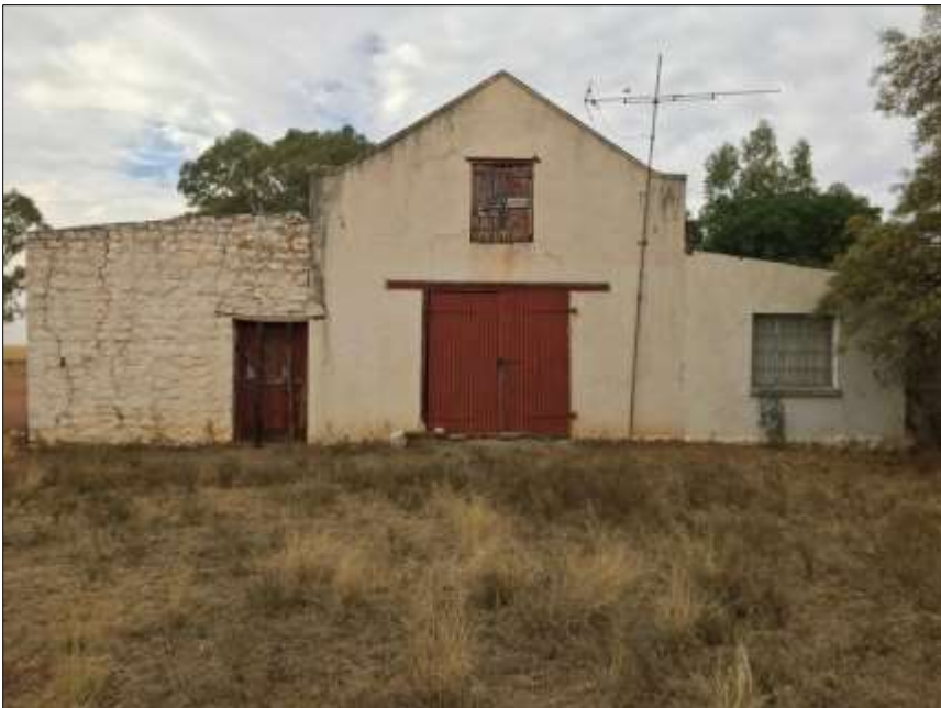
Figure 21. Back of the farmhouse. Note the later additions on either side of the building
