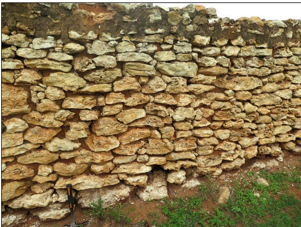
Figure 13: Calcrete blocks within the walls of the main ruined farmstead on Visserspan 40 (Hammer = 30 cm). These blocks provide good sections through the local calcrete hardpan in the search for bones / teeth / trace fossils and snail shells.
