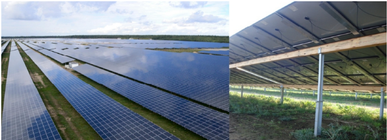
Figure 3: Typical single axis PV arrays
