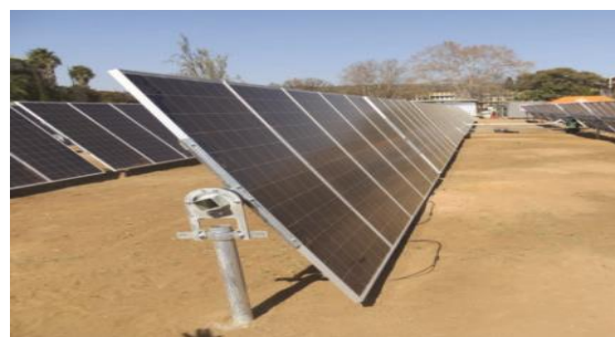
Figure 1: Single axis solar PV module tables raised 500mm above ground level (to a maximum tilt height of 3m). Proposed associated infrastructure includes a fenced construction staging area, a maintenance shed, inverter-transformer stations on concrete pads, office buildings and maintenance shed/s, a switch panel for connection to the power grid, all within the 222ha site.
