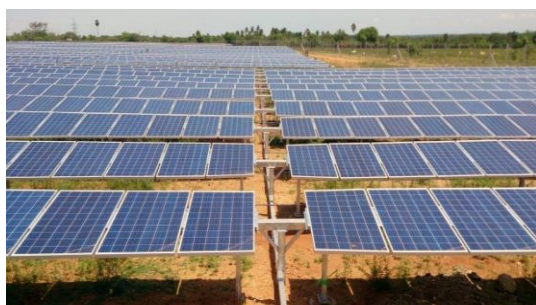
Figure 1: Single axis solar PV module tables raised 500mm above ground level (to a maximum tilt height of 3m). Proposed associated infrastructure includes a fenced construction staging area, a maintenance shed, inverter-transformer stations on concrete pads, office buildings and maintenance shed/s, a switch panel for connection to the power grid, all within the 222ha site.
