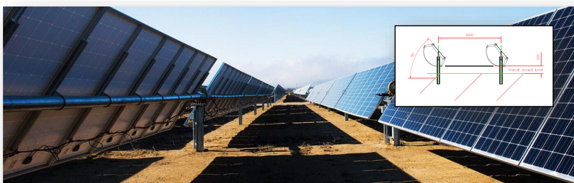
Figure 4: Single-axis vertical solar tracker system
