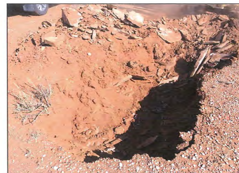
CONDITIONS OF HARD EXCAVATION IN QUARTZ-AMPHIBOLE SCHIST
