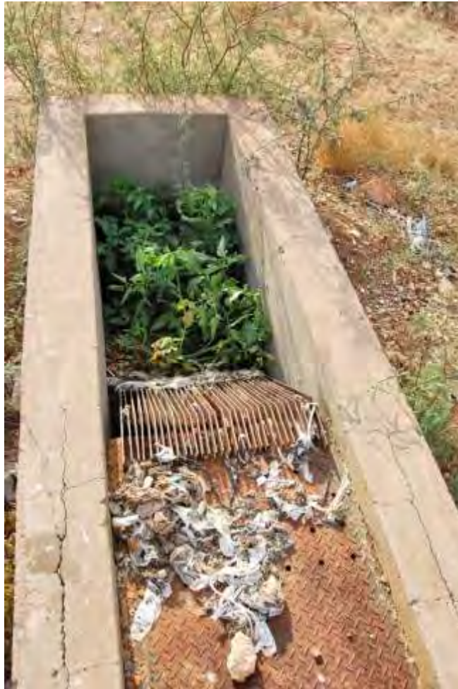
Figure 12 Intake structure
