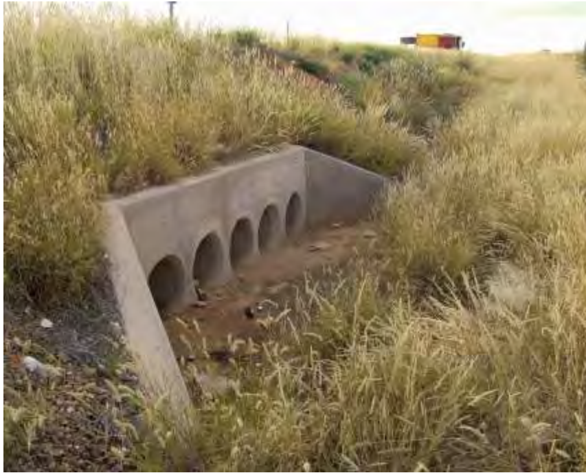
Figure 17 Culvert
