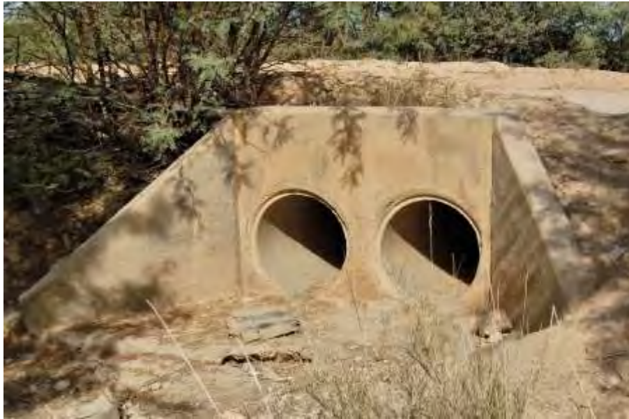
Figure 17 Culvert downstream of sewage pump station
