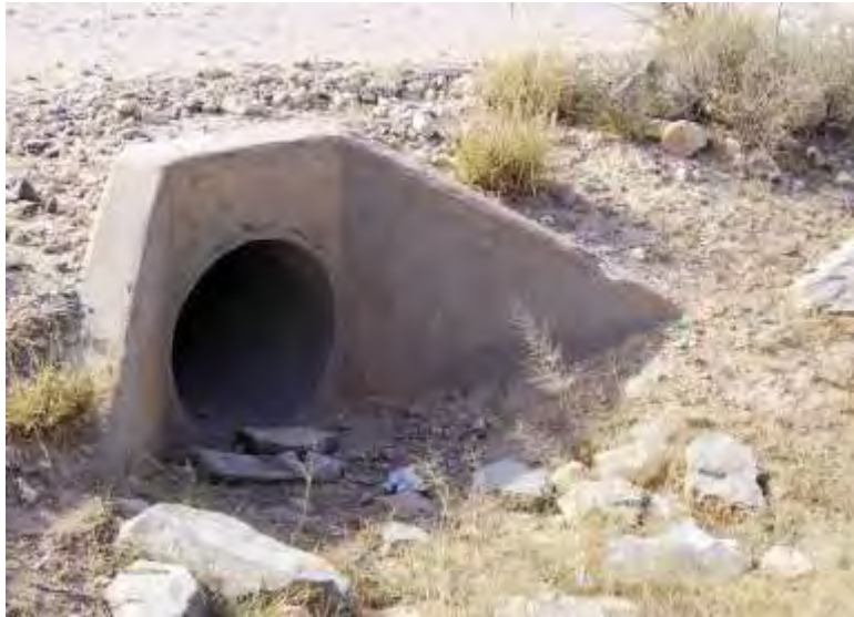
Figure 19 Culvert of longer drainage line
