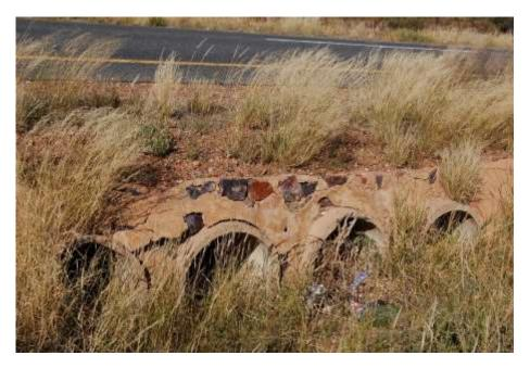
Figure 12 Pipe culvert
