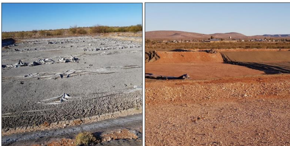
Figure 1: Oxidation dam systems at !Kheis Local Municipality (2019)
