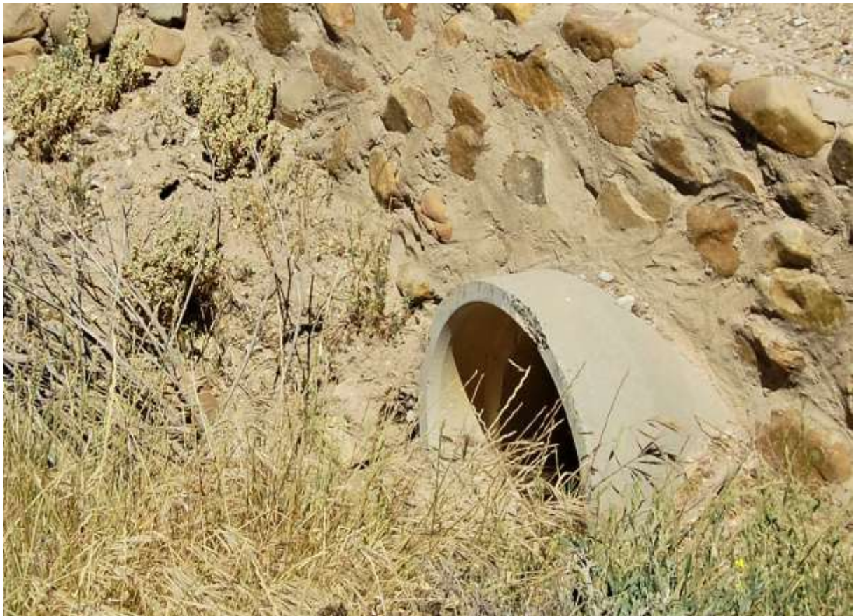
Figure 8 Sub-catchment 1 drainage line pipe culvert
