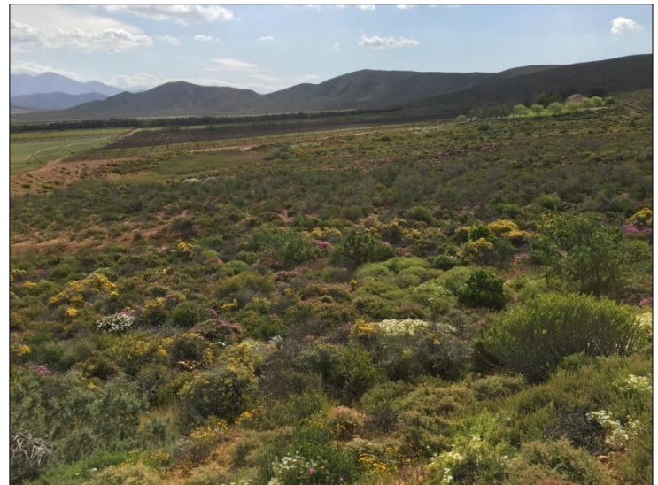
Figure 9. The abandoned dam site covered in dense vegetation. View facing west.
