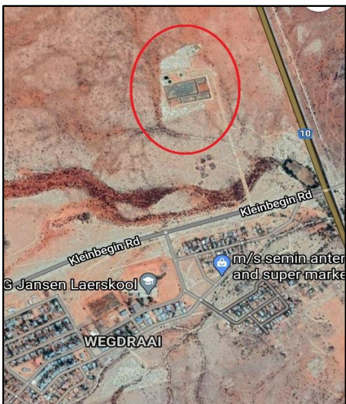
Plate 2: Wegdraai oxidation pond system in disrepair
