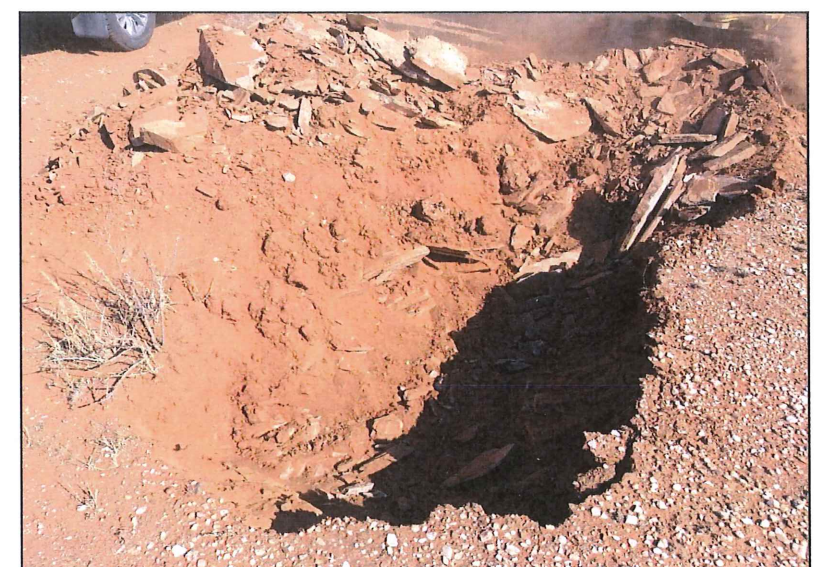
CONDITIONS OF HARD EXCAVATION IN QUARTZ-AMPHIBOLE SCHIST
