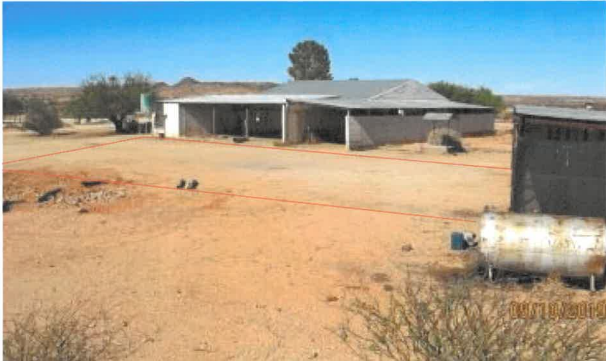
Figure 2: Looking from north-north-east, to south-south-east over the disturbed/brownfields site where the processing plant will be located (processing plant footprint outlined in red).
