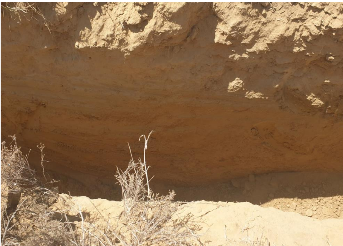
Figure 5-6: View of Test Pit 5 located in the dam basin for borrowing sand (upper soil horizon)
