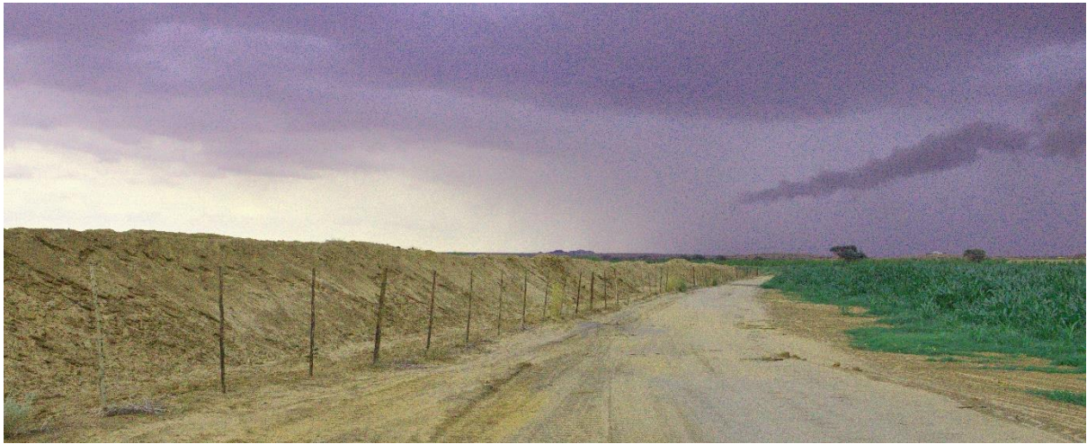
Figure 20 Berm on Hartbees River bank
