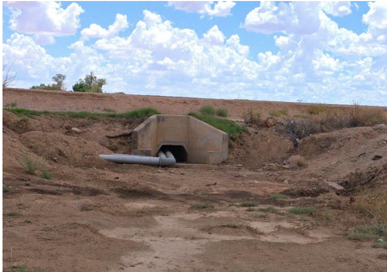
Figure 9 Pipeline crossing the irrigation canal
