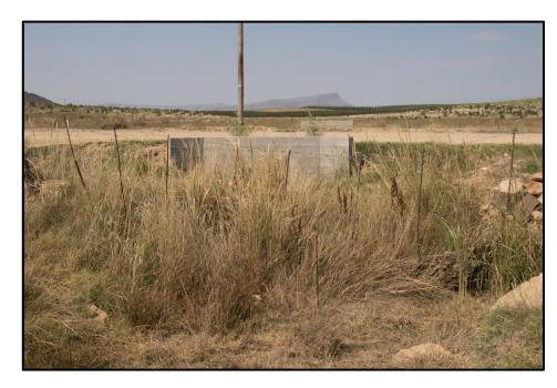
Figure 23. The culvert under the access road to the farm. Note the *Pennisetum macrourum* grass, typically found in wet situations.
