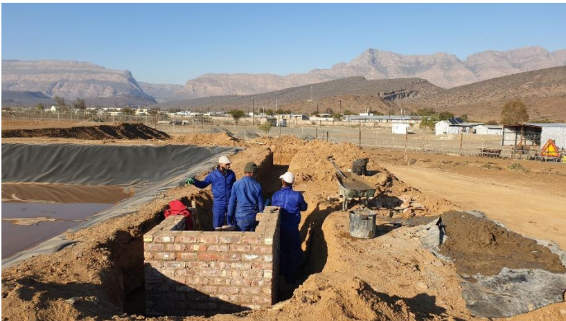
Cement mix on plastic
