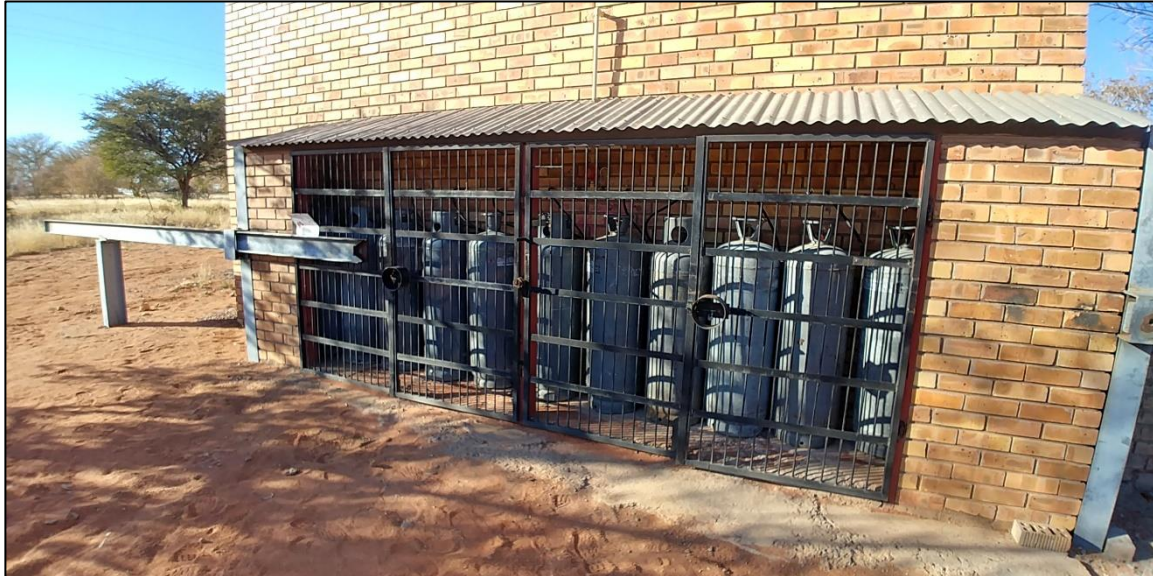
Figure 2. Liquefied Petroleum (LP) gas cylinders (48kg LPC/cylinder) were used for the cremation process. Six (6) gas cylinders are used at one time for each cremation.
