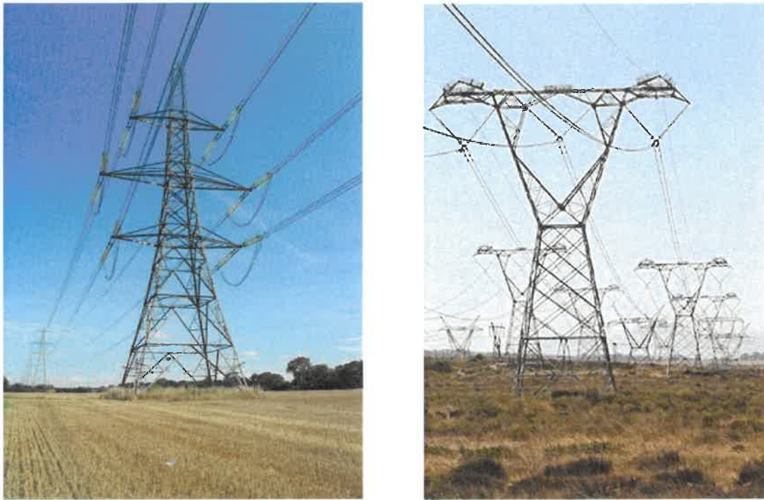
Figure 1: South African examples of the impact HV pylon footprints make on existing biodiversity whether it be cultivated lands/monocultures, or natural veld/grazing. A monopole structure would have proportionally less of an impact on the surrounding environment.
