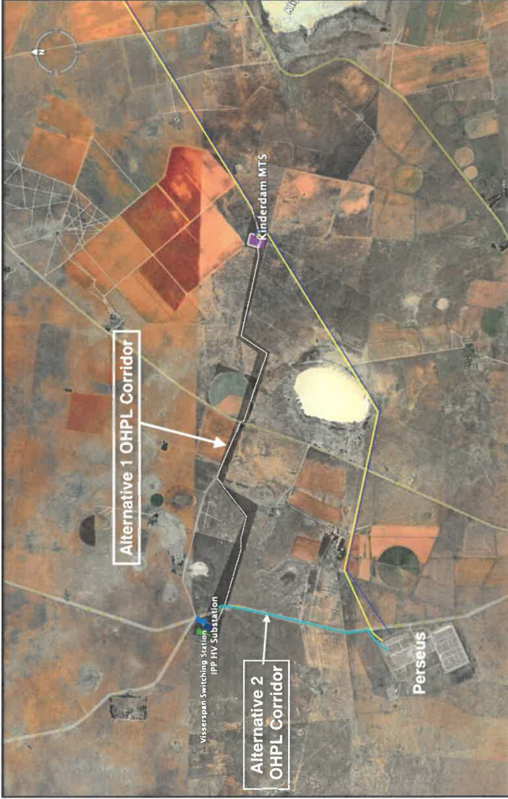
Figure 3. Google Earth™ aerial image showing the location of the Visserspan Switching Station, the Alternative 1 OHPL Corridor (black with white line), the location of the Kinderdam MTS, the Alternative 2 OHPL route (light blue line) and the Perseus substation. The yellow line between Kinderdam MTS and Perseus represents existing transmission lines.
