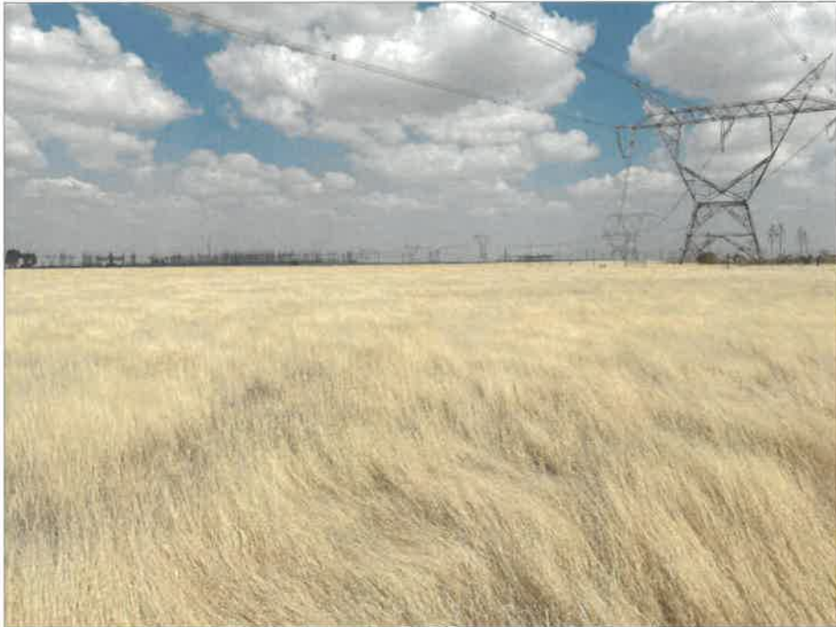
Figure 27. Proposed potential alternate powerline route on the Farm Walkerville. View facing south. Note the Eskom Perseus substation in the background of the plate
