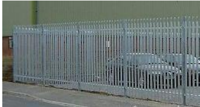
Figure 6: Typical galvanized palisade fence
