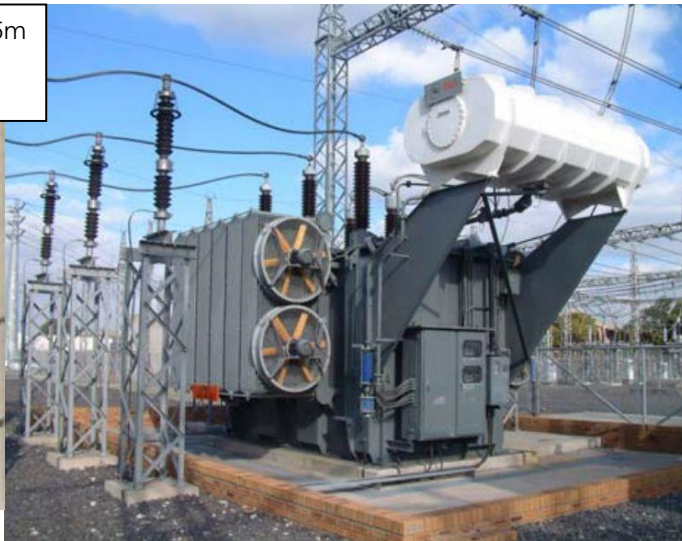
Figure 8: Transformer Pads and typical transformer
