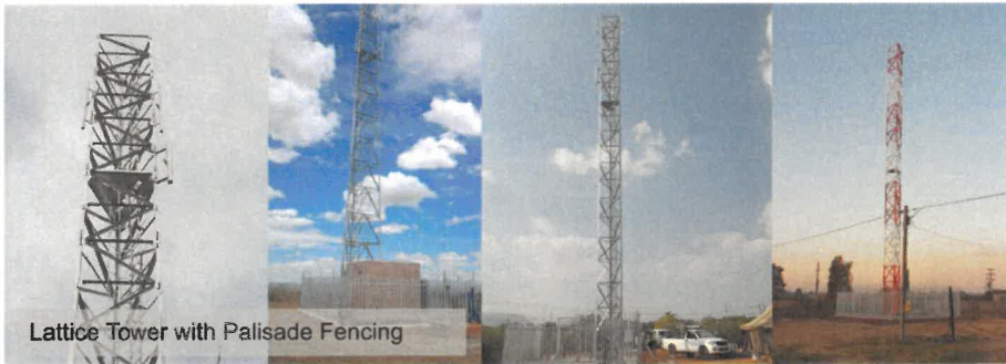
Figure 10: Examples of lattice tower with palisade fencing
