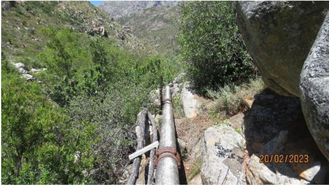
Photo 3: View of aboveground part of existing pipeline on rocky mountainside
