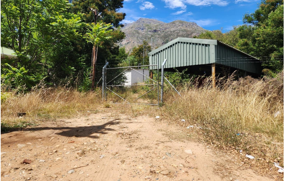
Photo 5: View of Wittebrug WPP where the water supply proposed pipeline ends
