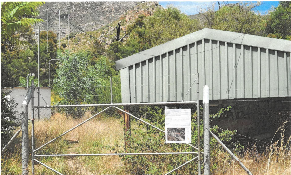
Photo 3: View of public notice placed on gate at Wittebrug WPP
