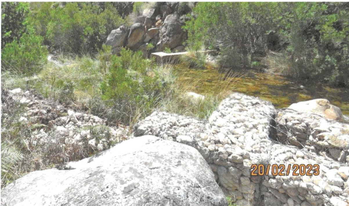
Photo 2: View of gabions at the weir where the intake point in the Teirhokskloof Stream is located
