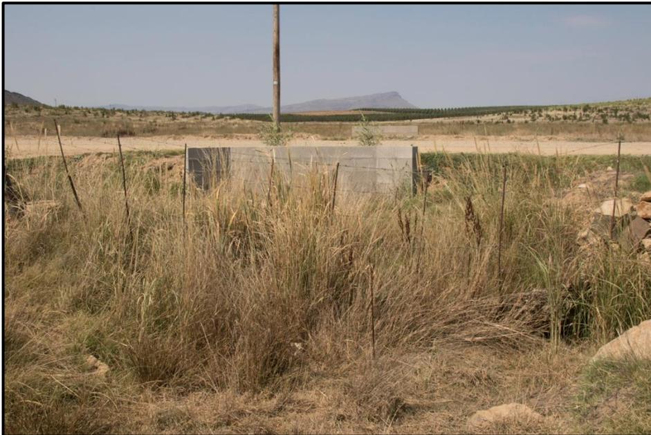
**Figure 23.** The culvert under the access road to the farm. Note the *Pennisetum macrourum* grass, typically found in wet situations.
