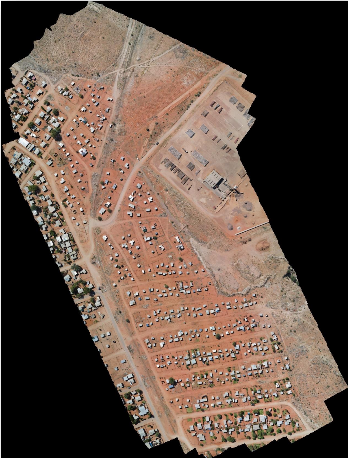
Figure 4: Street and Infrastructure - Pabalello Development Site 2
