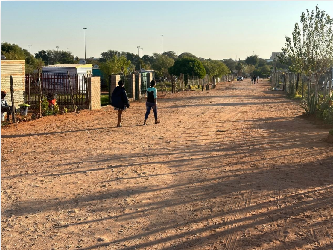
Figure 5: Street and Infrastructure - Pabalello Development Site 2
