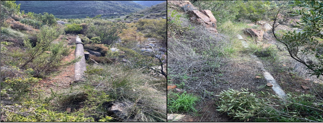
Plates 2a and 2b: Where the existing pipeline is buried or partly buried such as in these sites it should be left in place to prevent erosion.
