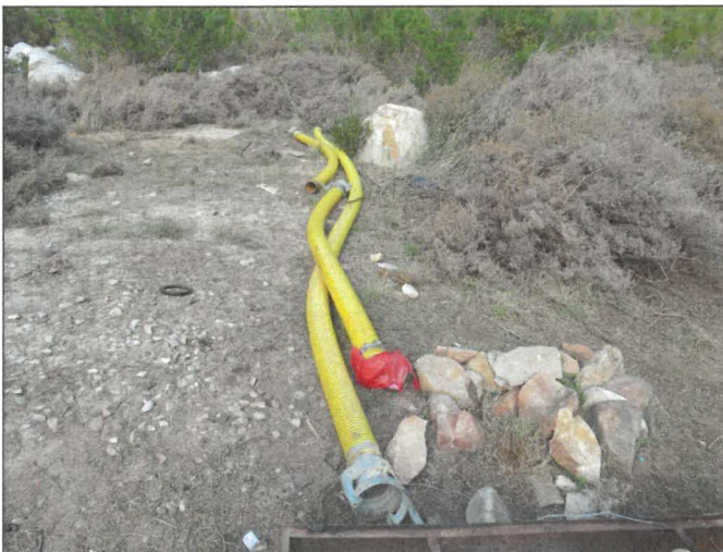
Plate 4: Discarded pipes and "braai" observed near the weir. Broken pieces of cement/asbestos pipe were also observed along the trail.
