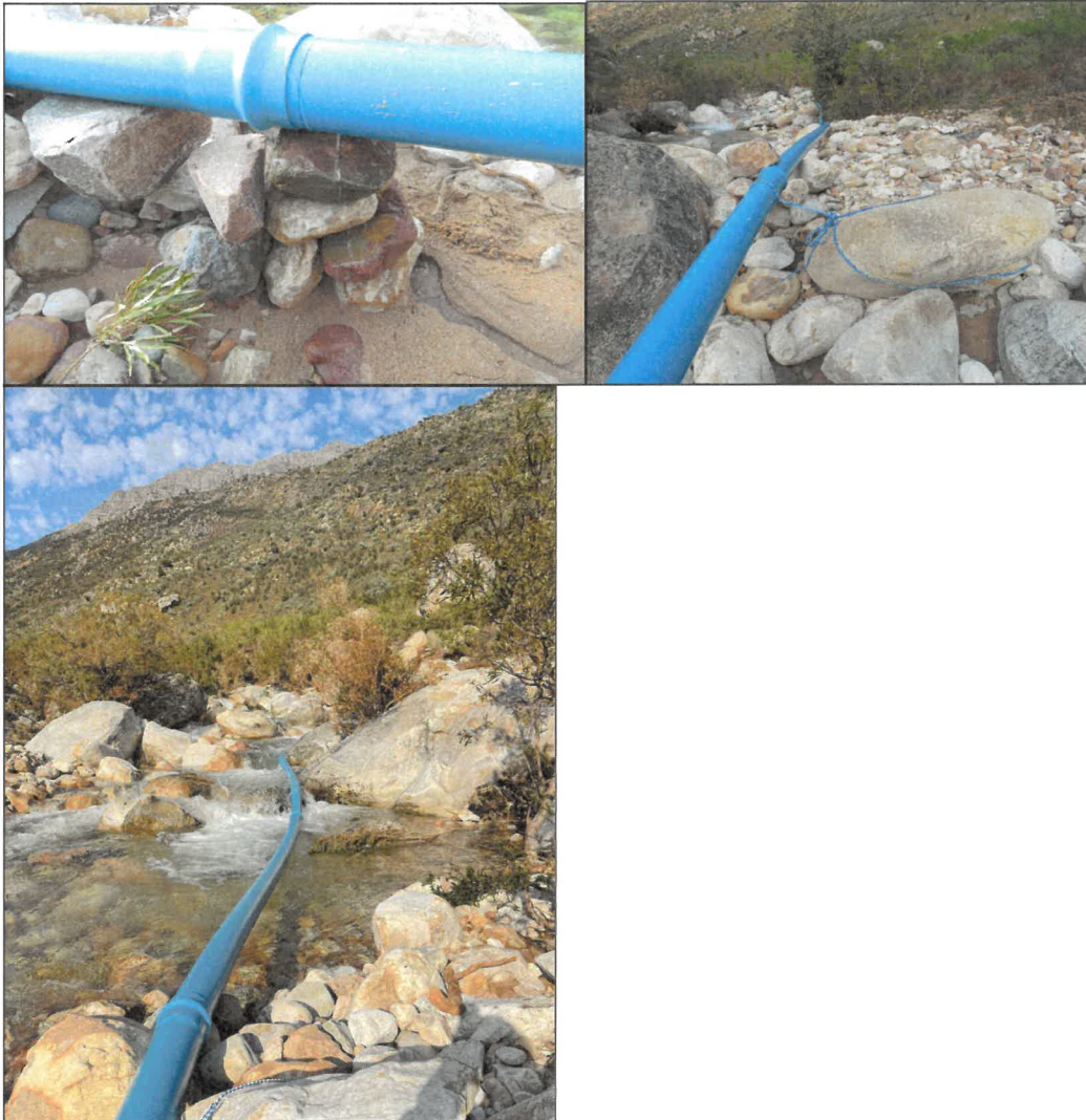
Plates 1a, 1b and 1c: Photographs near weir of blue plastic pipe which is precariously placed and needs to be replaced with a pipeline that blends into the environment. It is not clear when this blue pipeline was installed.
