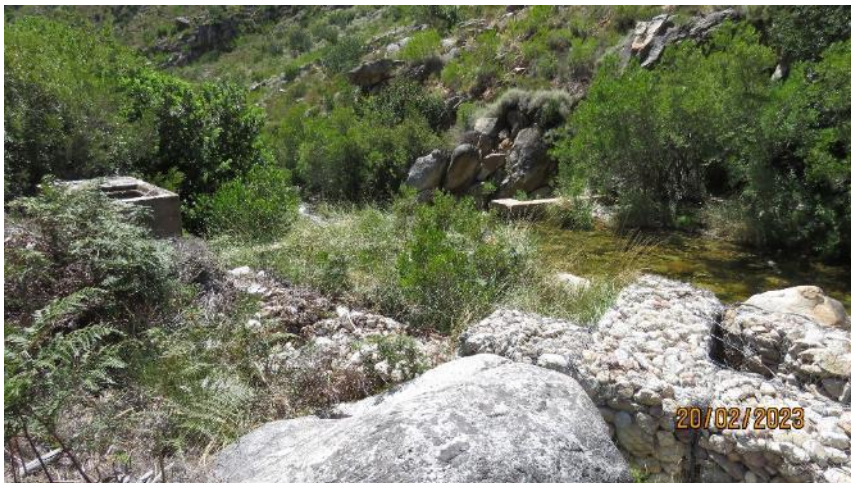
Photo 2: Looking downstream onto the inlet weir, which was placed in a narrow spot within the river.
