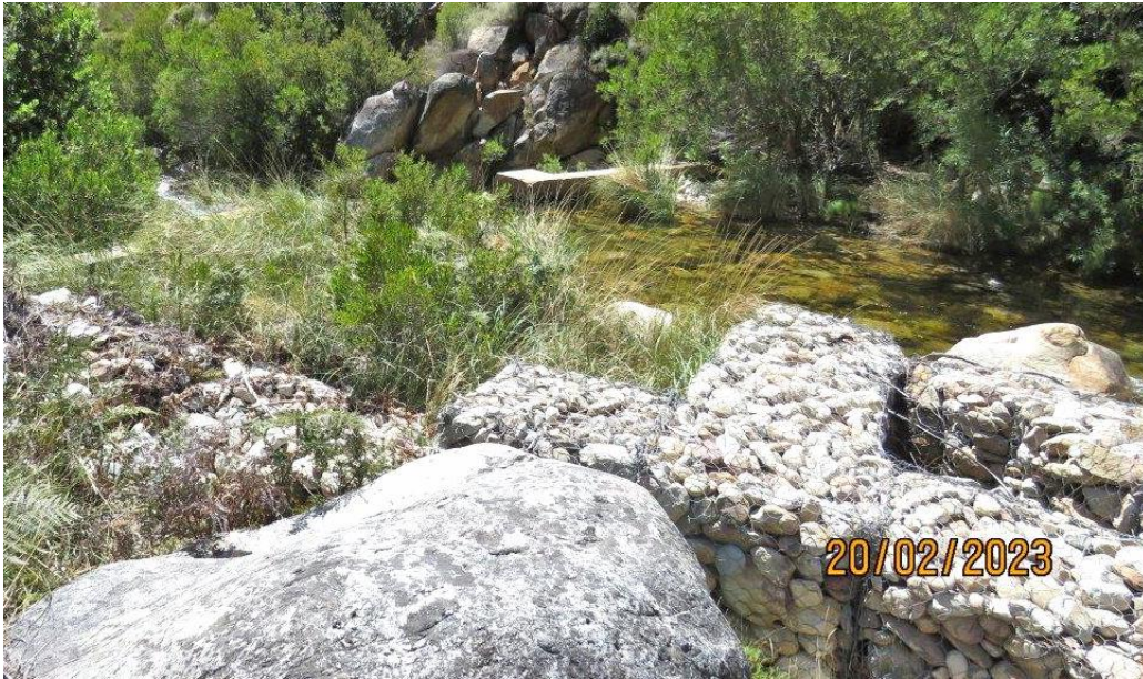
Figure 8 Gabions at the Tierhokkloof weir (Photo Peet Botes)
