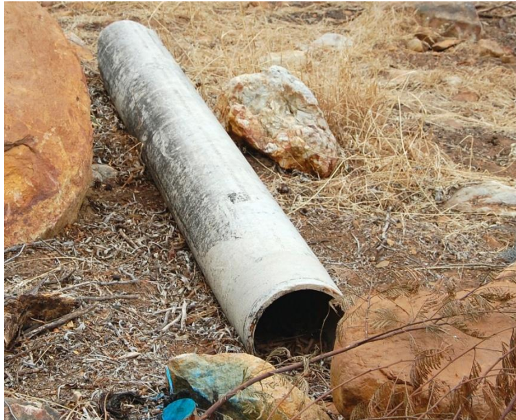
Figure 9 Broken section of pipe
