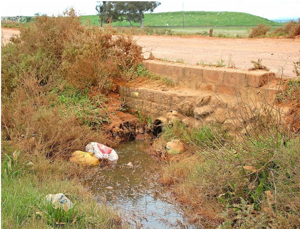
**Figure 13** Pipe culvert
