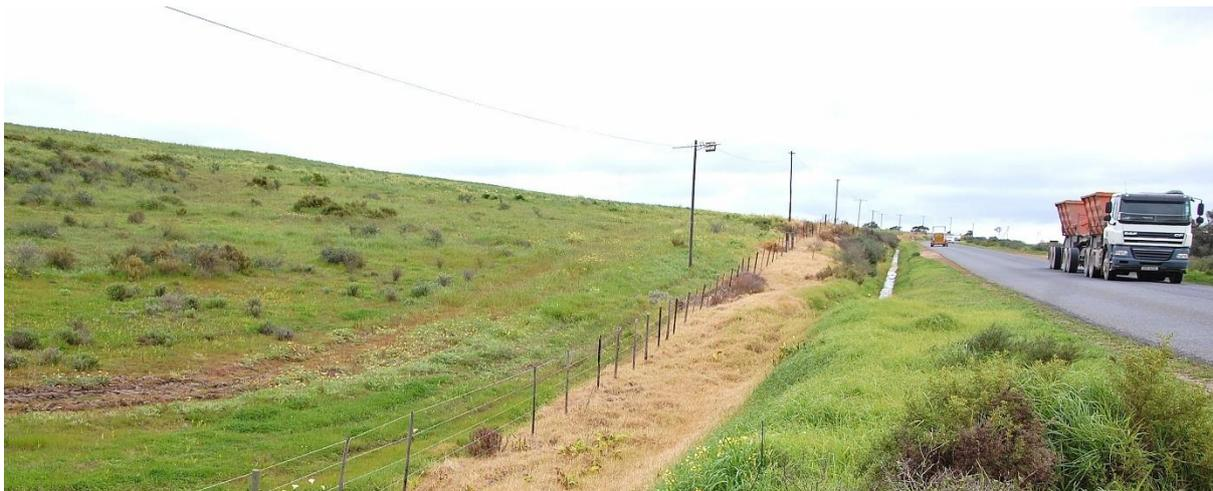
**Figure 11** Road drainage trenches
