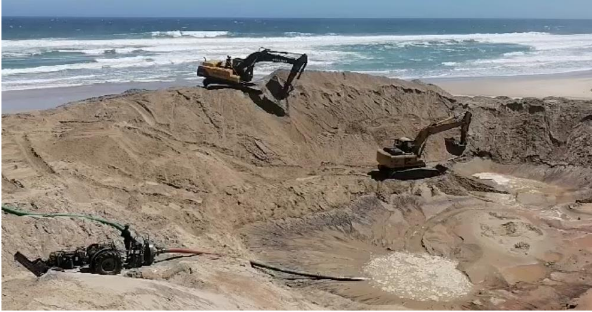
Photo 1: Berm to prevent waves from entering excavation
