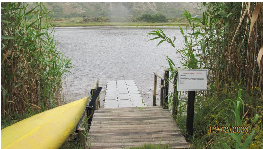
Photo 11: The small floating jetty on the edge of the Duivenhoks River.
