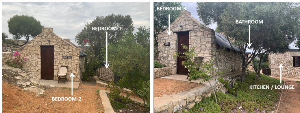
Figure 4: PHOTOS SHOWING BUILDINGS
