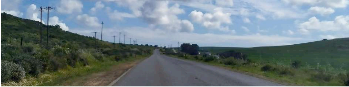
Photograph 4-20: R307/Darling–Yzerfontein Road view series: approaching Alexanderfontein .
