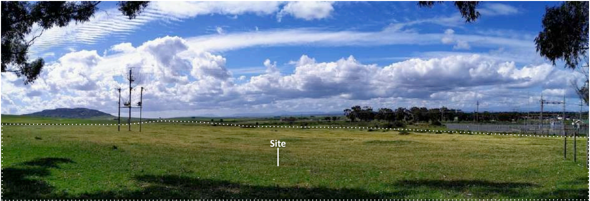
Photograph 4-11: R307/Darling–Yzerfontein Road view series: pasture and sub-station.
