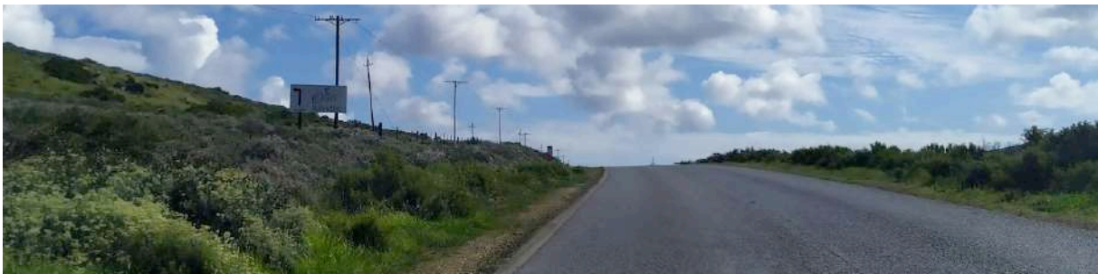
Photograph 4-19: R307/Darling–Yzerfontein Road view series: leaving the site behind.
