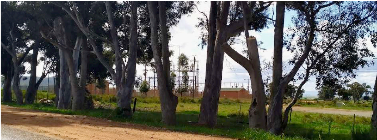
Photograph 4-6: R307/Darling–Yzerfontein Road view series: substation on site corner.
