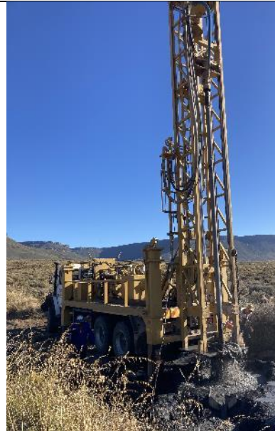
Borehole development at MAR 5.
