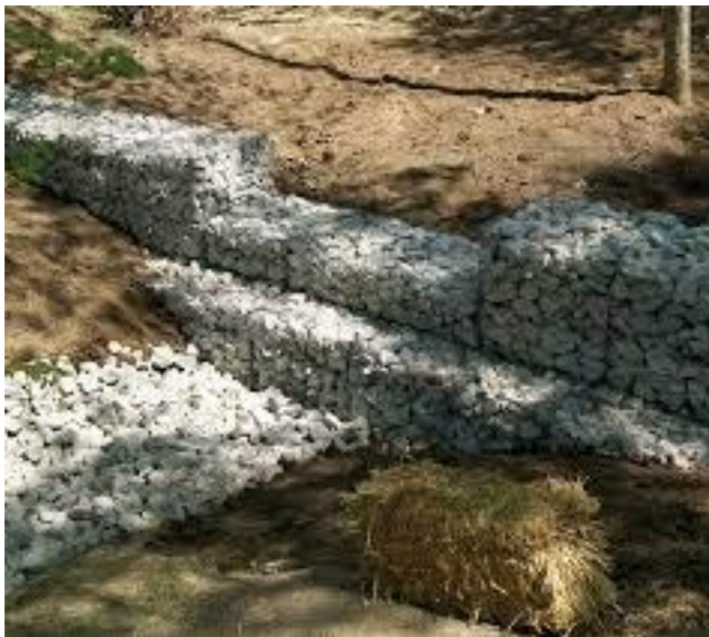
Figure 7: Typical rock filled gabion check dam structure
