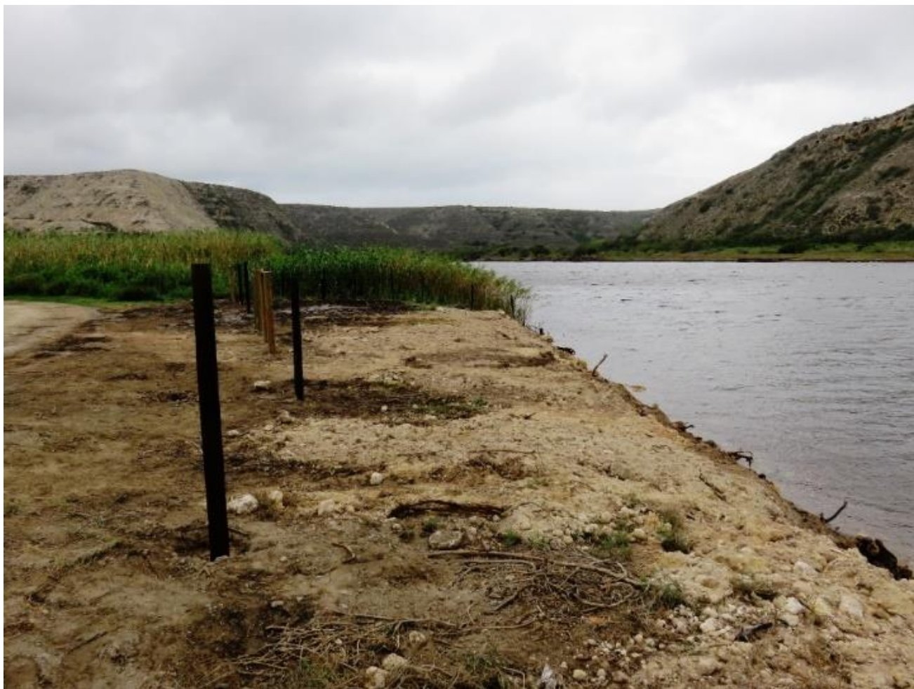
“new” river bank / Highwater “ecosystem 2020 – done be digger loader
