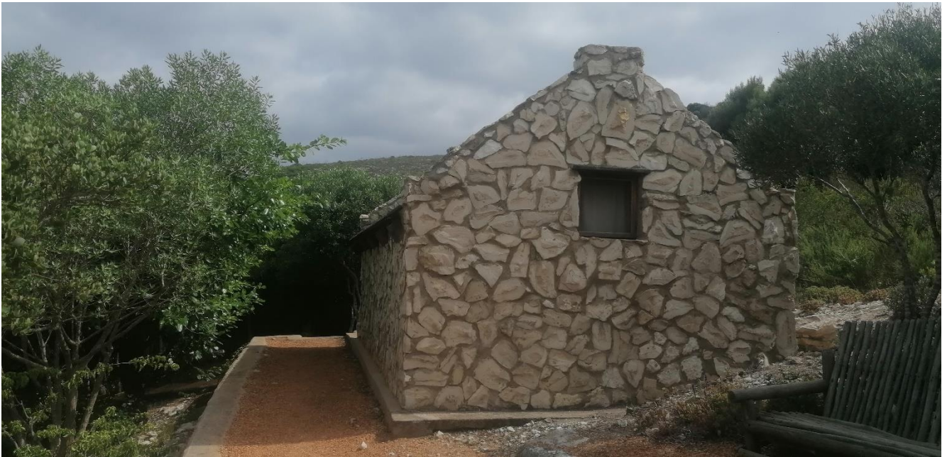
Figure 5. Site overview photographs of one of the bedrooms.
