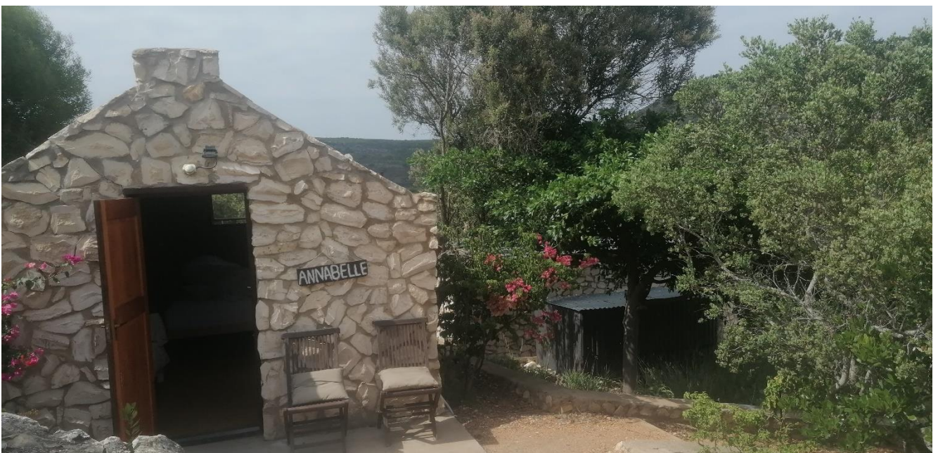
Figure 6. Site overview photographs of one of the bedrooms.
