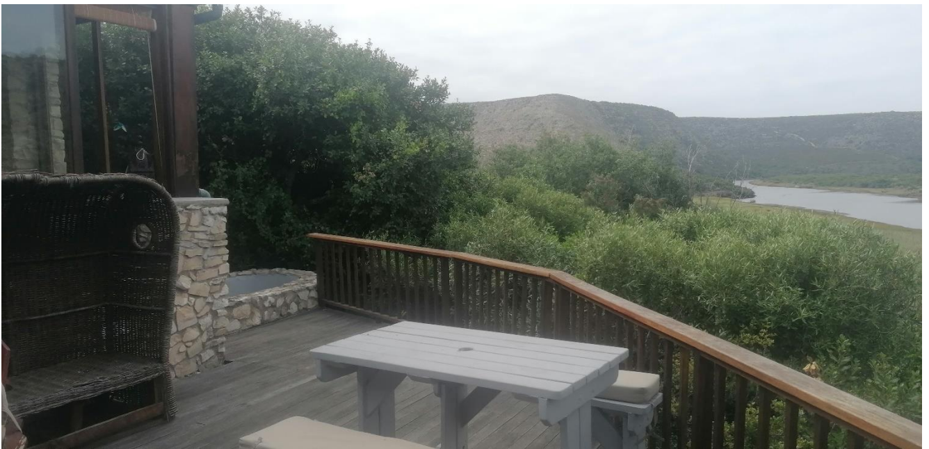
Figure 4. Site overview photographs of the main building area within the thicket vegetation.
