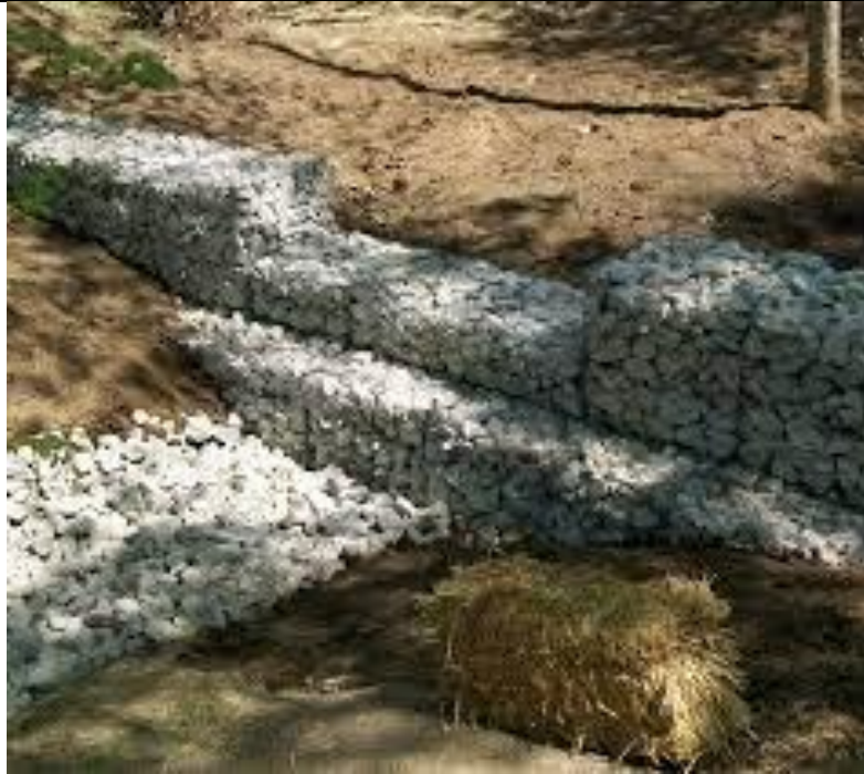
Figure 7: Typical rock filled gabion check dam structure
