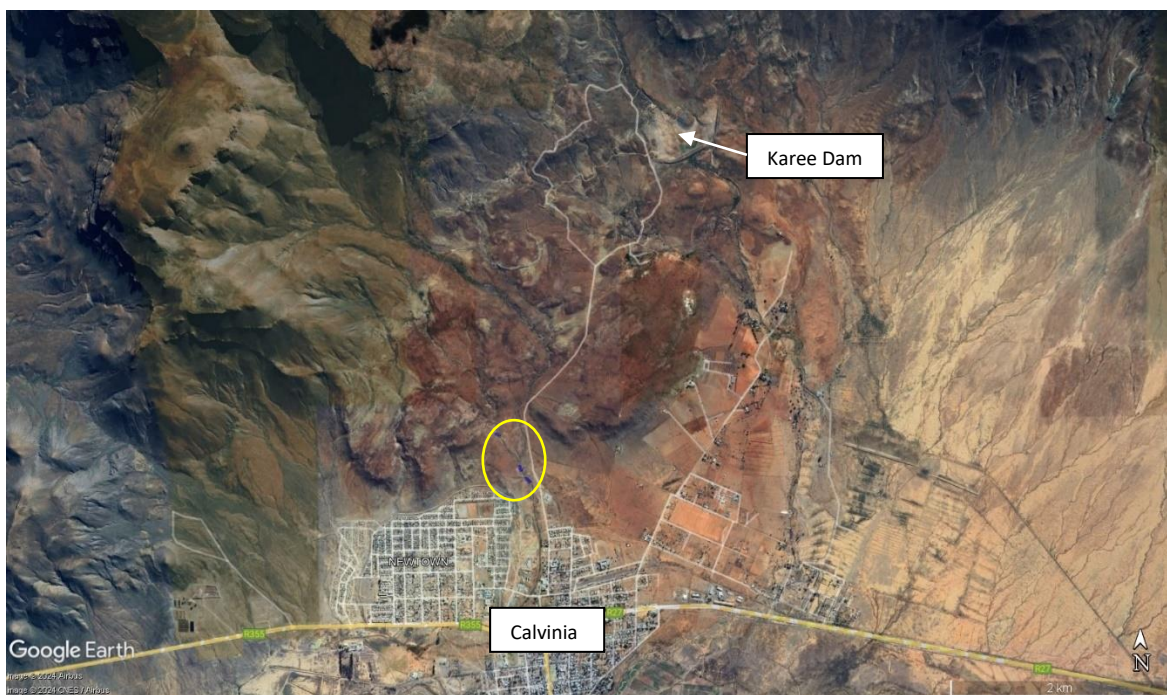
Figure 1: Location of Calvinia and the Karee Dam. Approximate location of the proposed project is indicated by the yellow circle.
